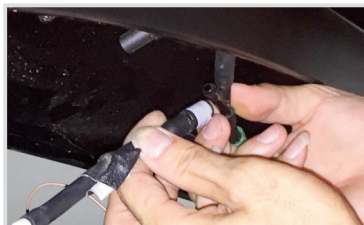
13. Take out the original joint of water pipe (Please be careful)
