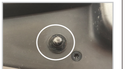
18. Dismantle the original tail door ball head
