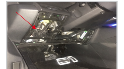
27. Dismantle the decorative plate
